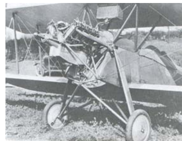
The Model 10 oleo-spring gear
