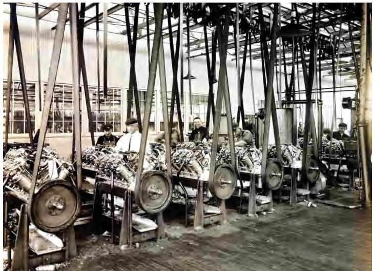
As we mentioned a couple of issues back, Willys manufactured OX-5 engines under contract for Curtiss to help fulfill the contract for Jenny aircraft during World War I. From what we understand, every engine built was tested with this equipment to show that they were properly assembled and fully functional before being installed in an aircraft.
