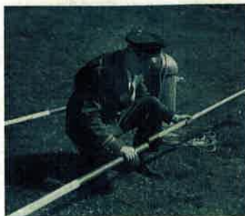
First step in erecting station is assembling two poles. Sections are joined easily.
