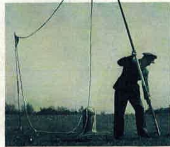
Transfer rope is strung necklace-fashion between poles. Attendant anchors second pole.
