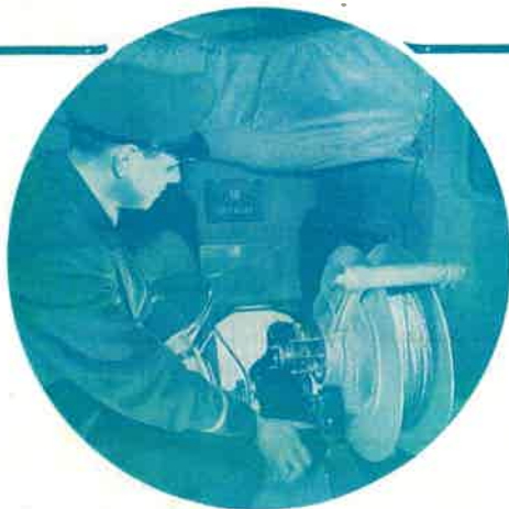
Plane's flight mechanic flicks switch, starting mechanism to reel container into aircraft in matter of seconds.
