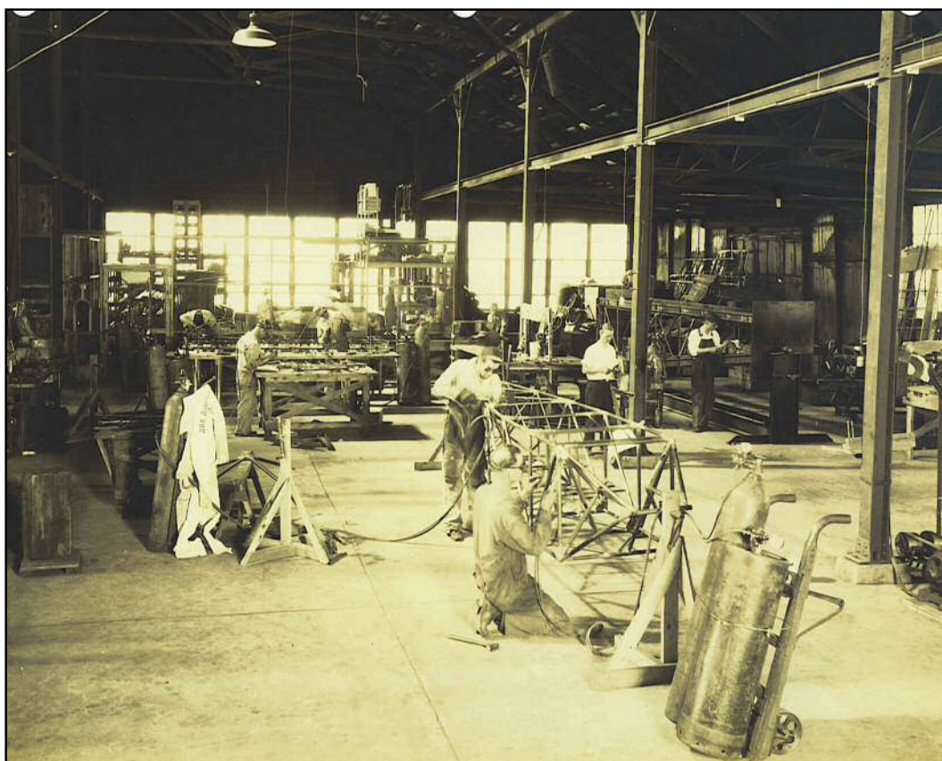
Above, welding fixtures designed by Al Vollmecke to facilitate exact duplication of welded structure. Upper photo is the rotating fuselage fixture and below workmen are welding on a fuselage frame that has just been removed from the master jig. The frame appears to be an OX-5 powered model 3C3. Note large oxygen and acetylene tanks and long hoses.
