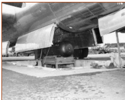
Loading Little Boy bomb on Tinian, using hydraulic lift.
