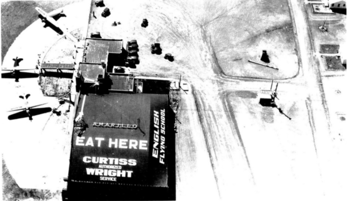
Aerial view of English Field Terminal late 1930's
