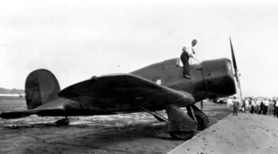
Jimmy Doolittle climbs out of the Lockheed 'Shelllightning' Orion 9C with a metal fuselage and retractable landing gear.
